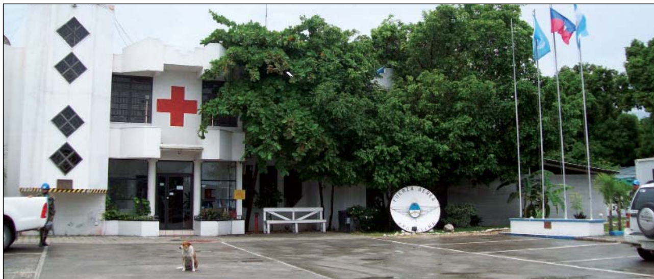
Argentine Hospital in Port-au-Prince (Haiti).
