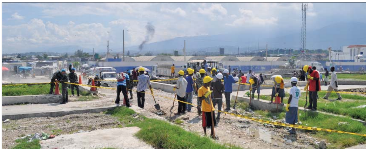
The beginning of work led by the Brazilian contingent in Place Fierté (Photo: courtesy of BRABAT I, Haiti).
