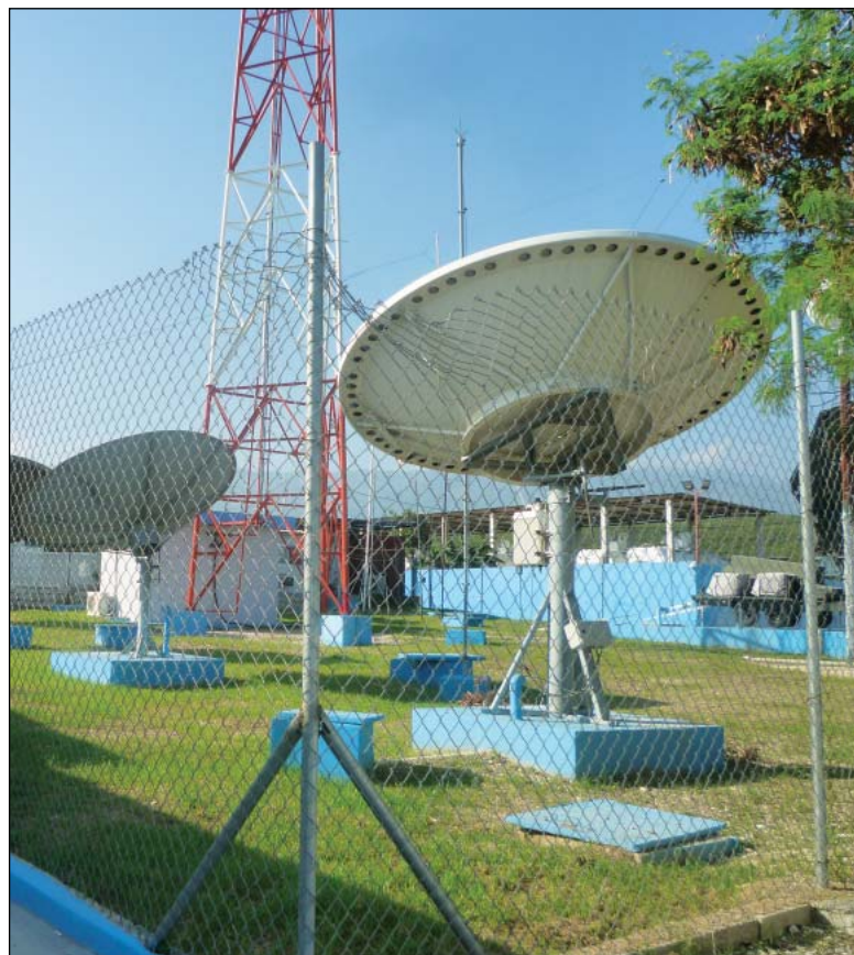
Telecommunications installation, BRABAT I (Haiti).
