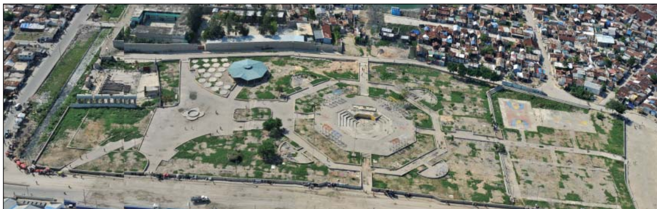
Aerial view of Place Fierté, Cité Soleil (Photo: courtesy of BRABAT I, Haiti).
