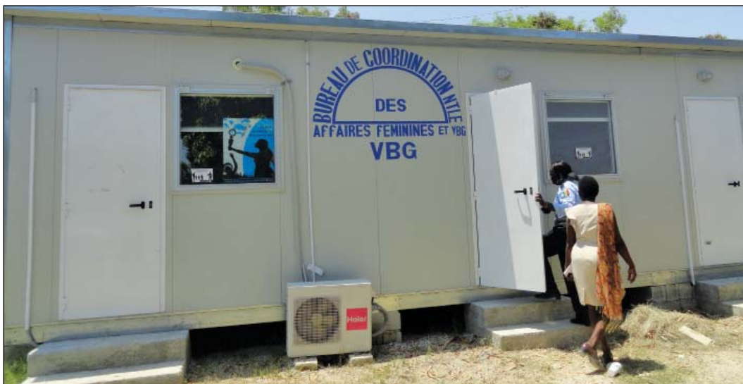
Location of the HNP National Coordination Office for Gender at the police quarters, constructed by the SGBV project (Haiti).
